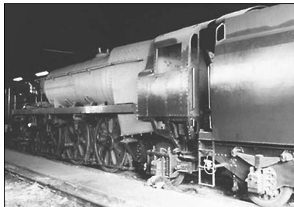
No.34059 undergoing restoration at Sheffield Park. Photo: Richard Salmon
